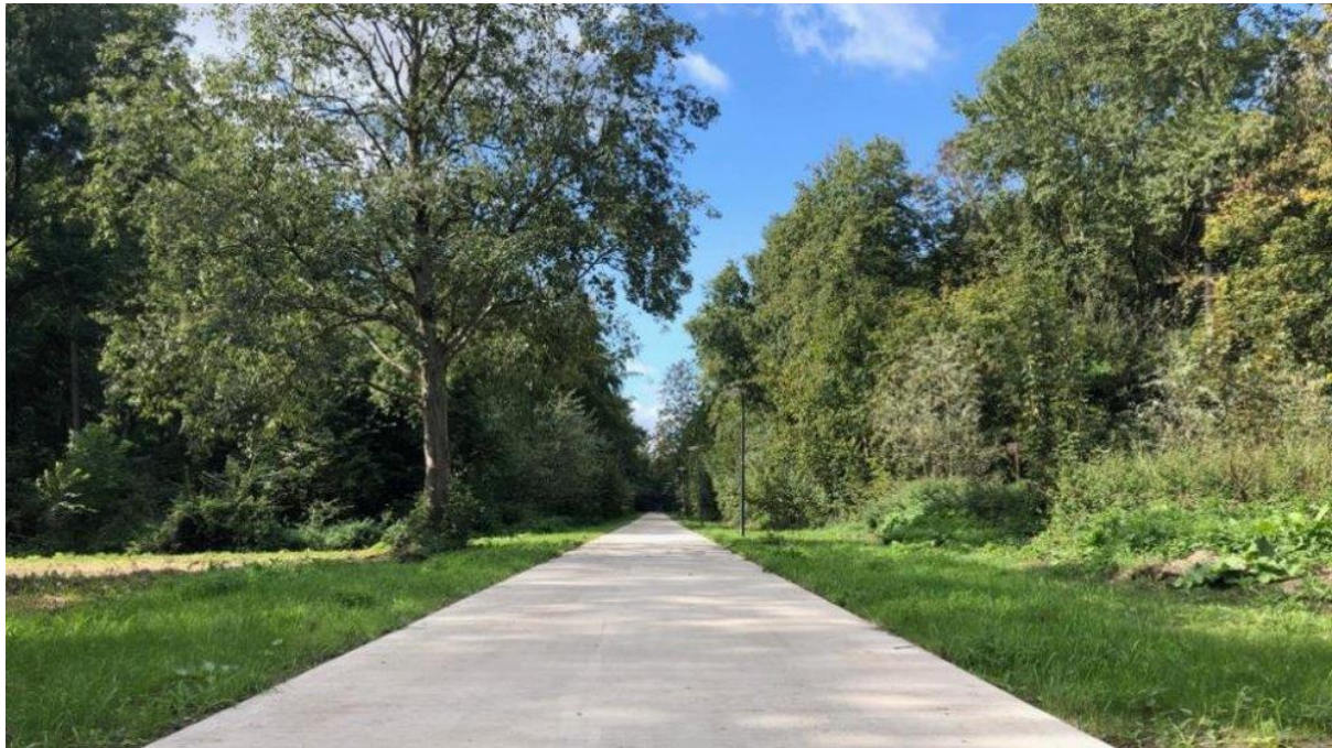
Figure 2. Example of green concrete in Almere
